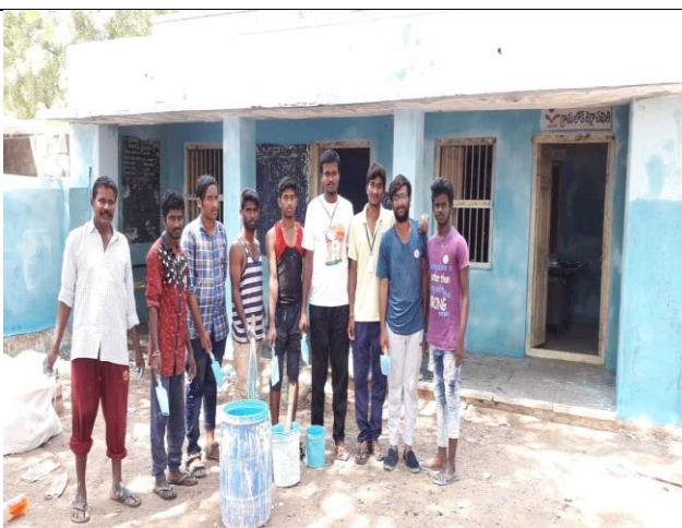
WALL PAINT TO THE GRAM PANCHAYATH OFFICE
