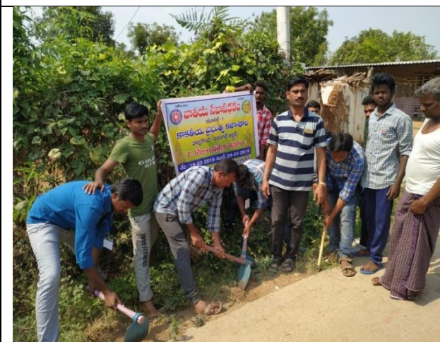
SIDE DRYNAGE CLEANIG
