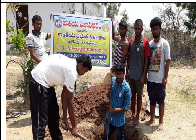
DIGGING OF SANITARY PITS
